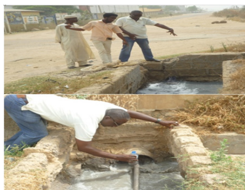
Figure 10. Stinking open drainage in the study area at sample collection point.
